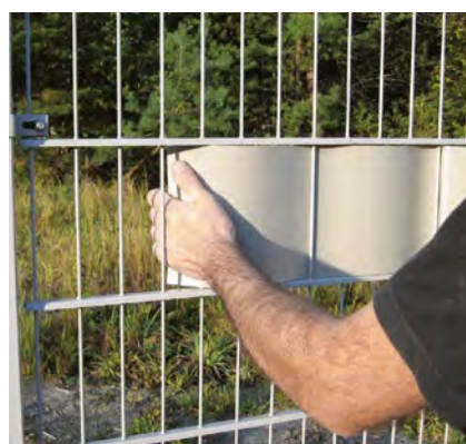
The fence strips mounted on the fencing panels.
